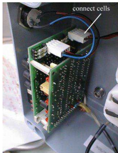
Photo 5.1b. Connecting the batteries
